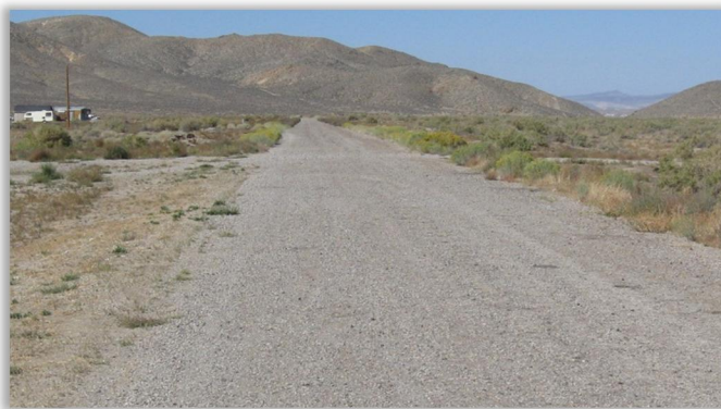
US 50, Near Middlegate, existing parallel gravel road
