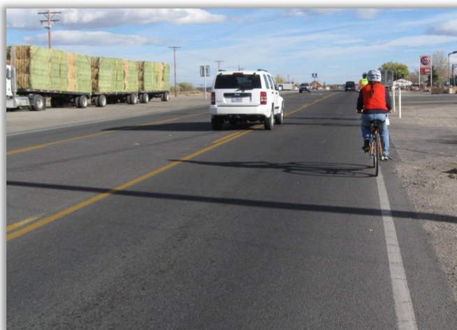
US 50 (Old Lincoln Highway/E Main Street), Fernley: Narrow shoulder
