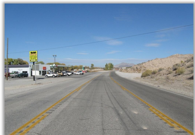
US 93 in Alamo: Widening for turn lanes can result in no shoulders.
