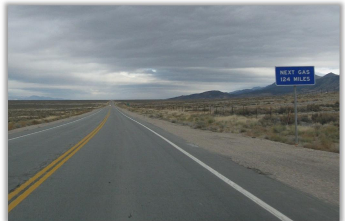
US-93, North of Ely: Certain areas of Nevada currently have very long distances without any rest stops or water.
