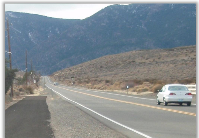
Jacks Valley Road, Minden: Narrow shoulder and path near roadway
