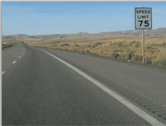
I-80: Although there is a rumble strip located adjacent to the fog line, wide shoulders provide adequate space for bicycles along this route.
