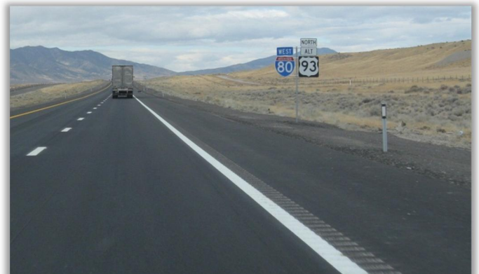
I-80: Segments of I 80 have rumble lines, with the rumble strip under the fog line, which maximize the space available for bicyclists while also serving as a safety measure for motorists.
