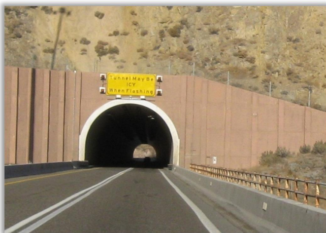
I-80 at Carlin Tunnel, Narrow shoulder entering and in tunnel
