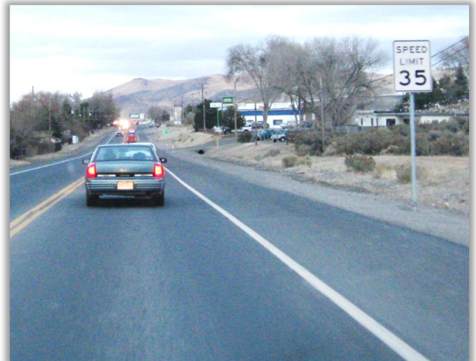
SR 535, Elko: A wide shoulder through this rural community serves as a bicycle facility as well as a break down area for vehicles.
