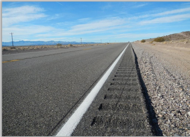
US 95, South of Goldfield: Rumble strips placed within a narrow shoulder make the shoulder unusable for bicyclists.
