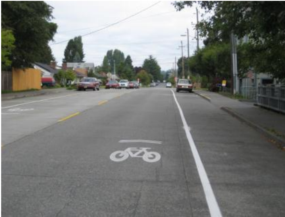
Figure 5 – Marked Shared Lane Facility
