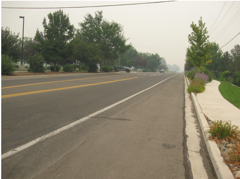
Figure 6 – Paved Shoulder Facility
